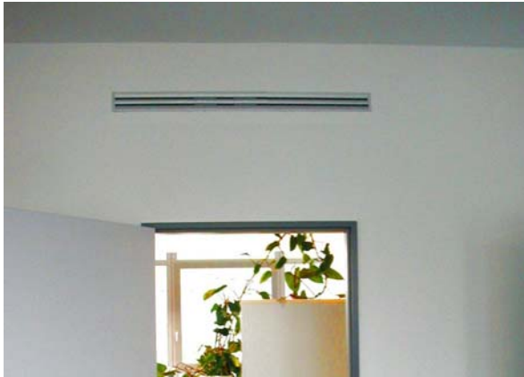
Installation example Type LDK-B with two slot rows
