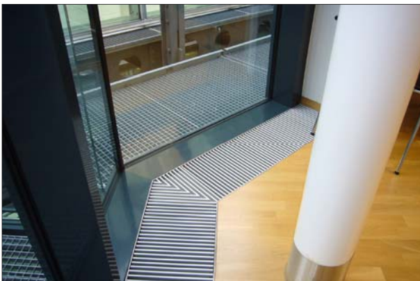
LTG fan coil unit type VKB - installation example
